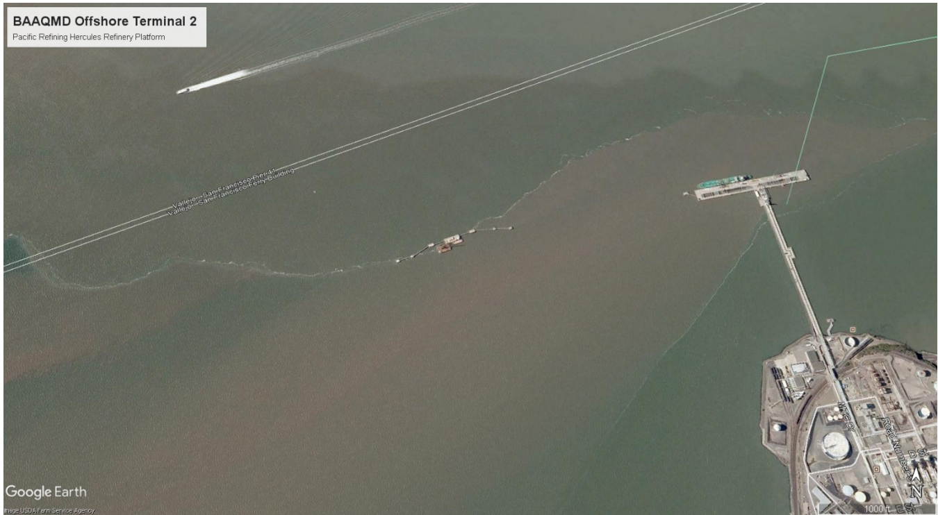
Figure 3-6. Marine Loading from Pacific Refining Hercules Fixed Berth
